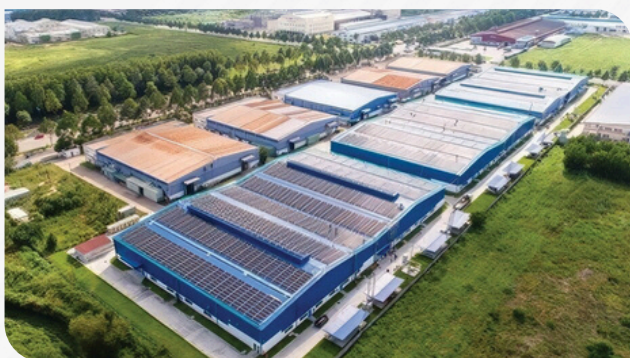
New CC Rental Factory Construction
